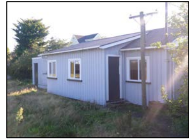
Former croquet club building in Blighs Garden
