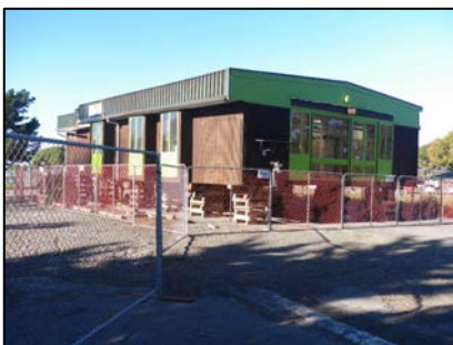
Transitional community building being put into place
