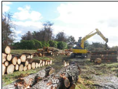
Tree removal in Bridge Reserve 2012
