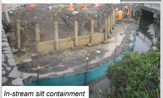
Silt containment on Warden Street
