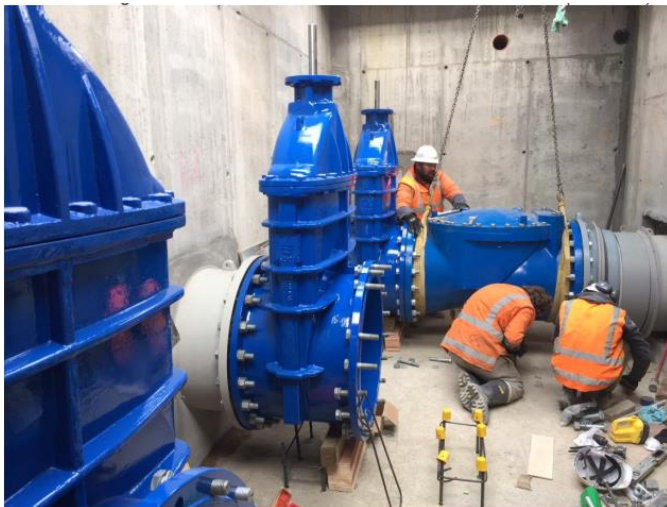
Mechanical equipment being installed
