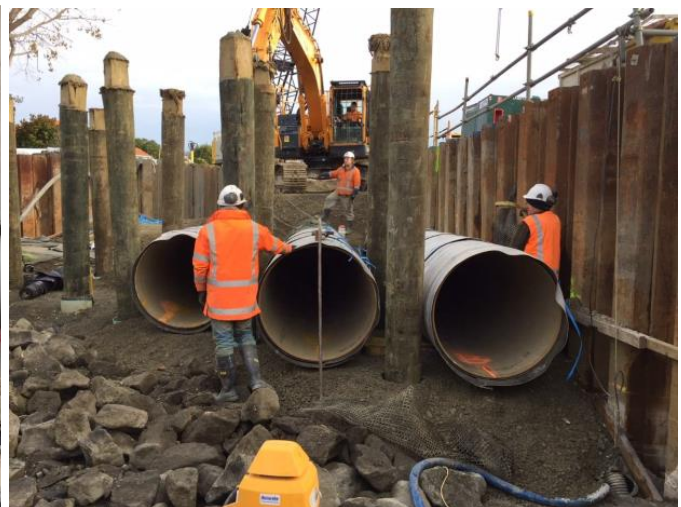
Outfall structure and wharf under construction
