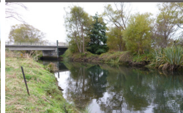
SITE 48: Styx River at Kainga Rd (looking upstream from bottom of site)
