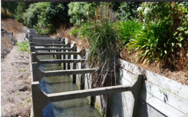
SITE 12: Horners Drain at Hawkins Rd (looking downstream from top of site)
