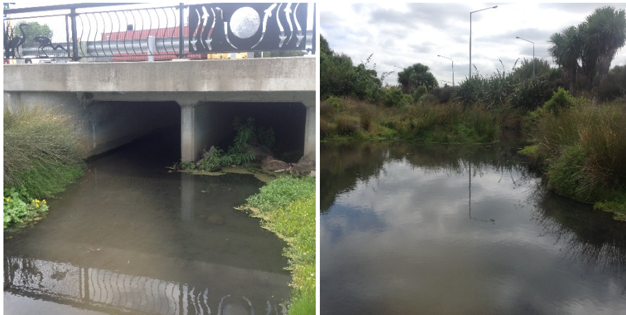
Photo 18. City Outfall Drain / Linwood Canal (Site 18), looking downstream (left) and upstream (right).
