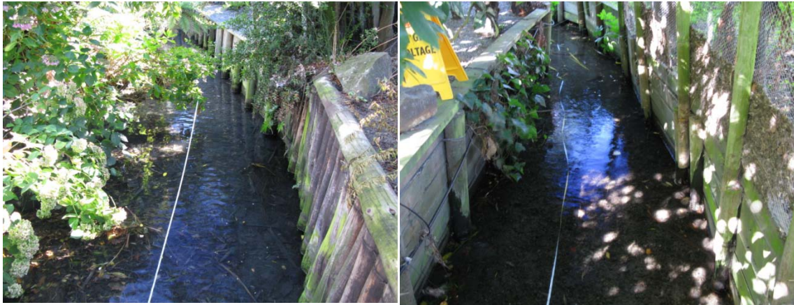
Waimairi Stream North Branch, looking upstream.
