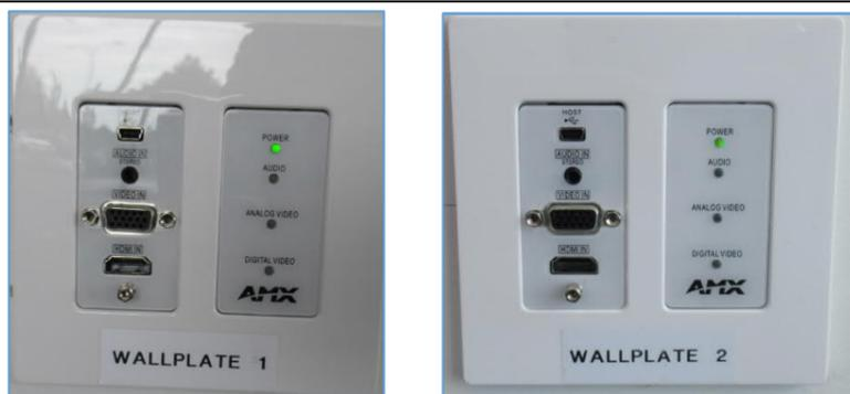
2. Locate the “Wallplate” under the TV Screen (Please note: this room has two “Wallplates” you can connect to. These are located under both TV screens) – “Wallplate 1” (kitchen end, west side) & “Wallplate 2” (near large fire exit doors, eastside)
