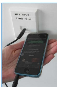
3. Connect the device to your 3.5mm cable and plug it into the "MP3 Wall Input Socket"
