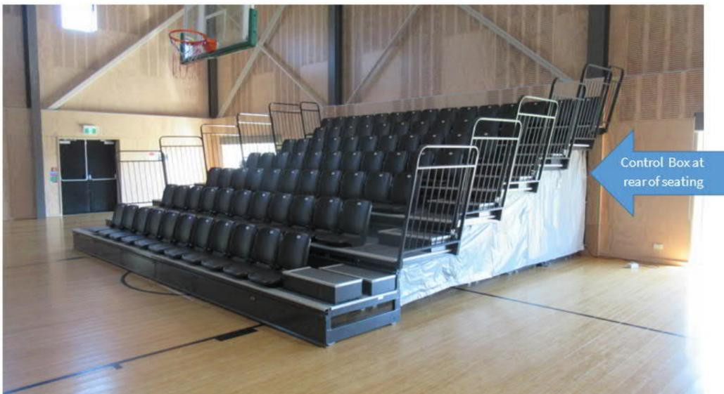
4. Locate the Control Box on the RH side rear of the Stadium Seating, behind the grey curtain. (The Handheld Pendant Control connects into this wall box)
