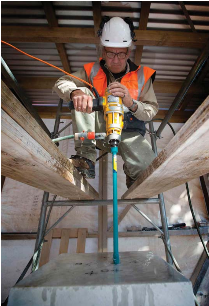
Sculptor Mark Whyte drills holes down into the replica marble leg for the carbon fibre rods that will strengthen the structure.
