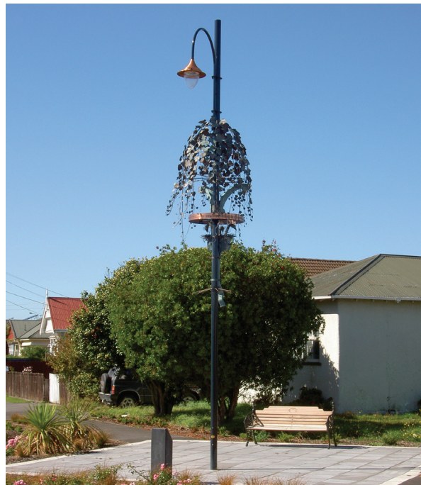
Using streetlight poles to display artworks (Spencer St)
