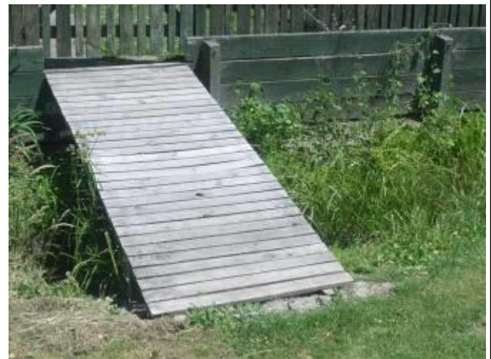
Wooden ramp with no handrails or non-slip surface. As this ramp leads solely to a private residence it is a privately owned ramp.
