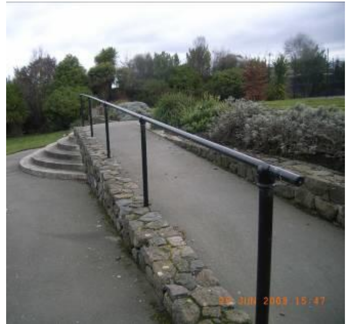
Asphaltic concrete ramp with handrails but no non-slip surface.
