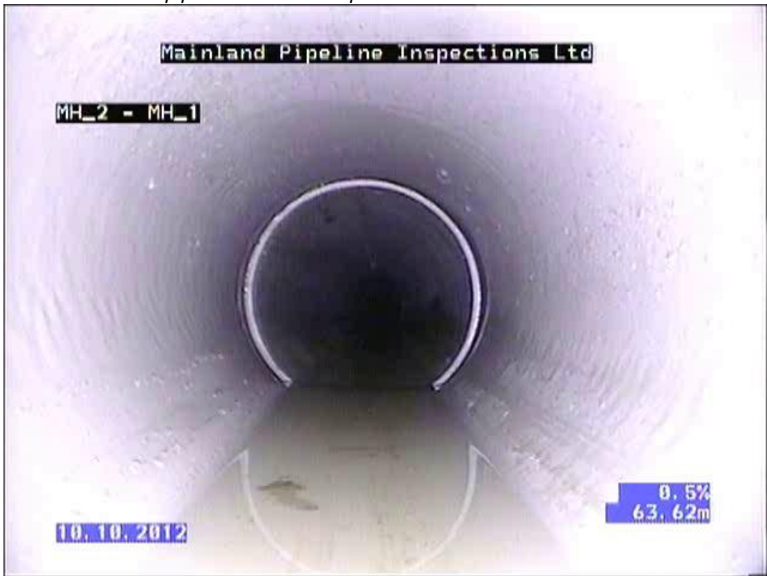
Photo 3: 300mm pipe with a 20 mm Dip
