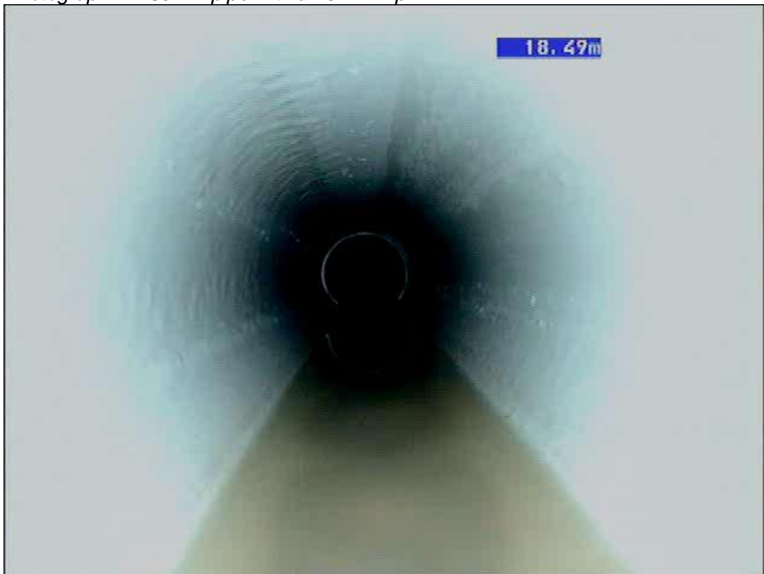
Photograph 1: 150mm pipe with a 20mm Dip
